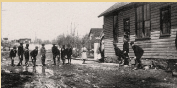
Lake Ariel One-Room Schoolhouse
